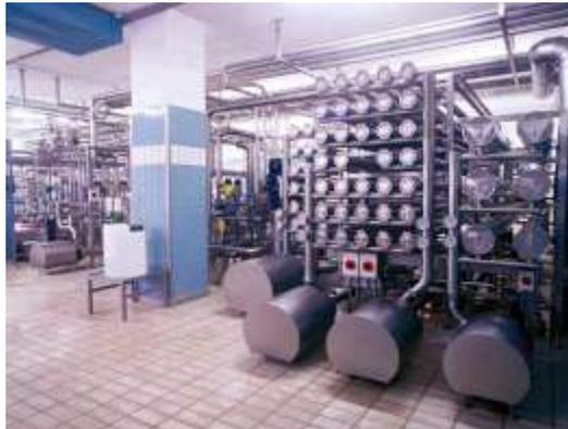
**Fig. 12.6 Integrated membrane filtration system comprising UF plant for WPC & RO plant for lactose concentration**
